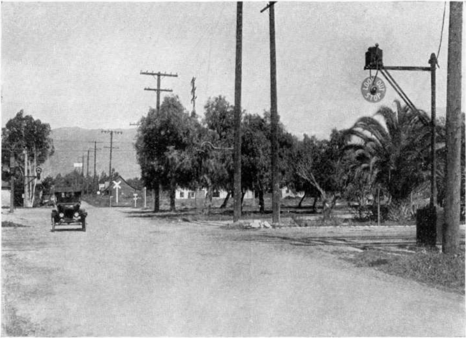
Magnetic Flagman installed at Claremont, California, on Atchison, Topeka & Santa Fe R. R. More than 300 in service on this railroad.
