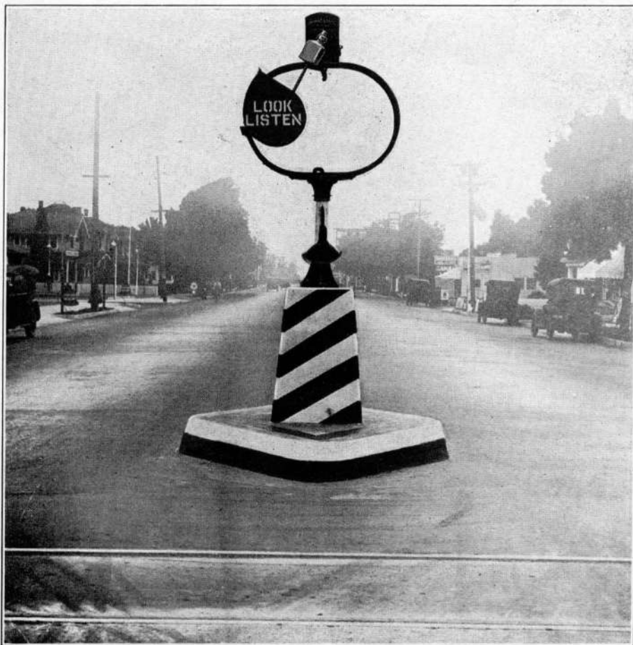
Center of Street Installation of Type LB-8 Magnetic Flagman (three position), on Union Pacific R. R. at Anaheim, California.
