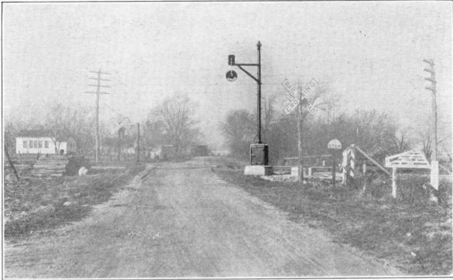
Installation of Magnetic Flagman (two position, lower quadrant), on the Atchison, Topeka and Santa Fe R.R. at Emporia, Kansas.
