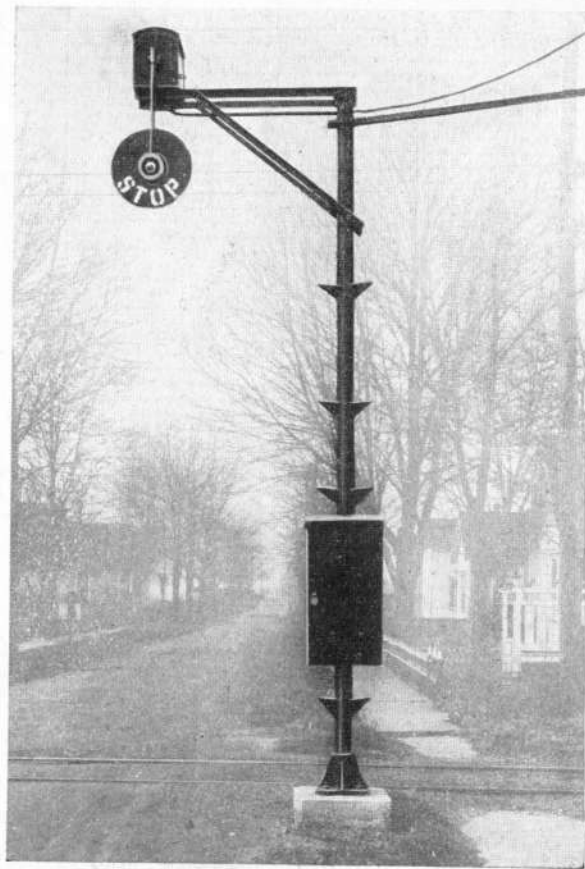
600-volt D.C. Electric Line Installation of Magnetic Flagman (two position, lower quadrant), on Interstate Public Service Co. at Scottsburg, Indiana.
