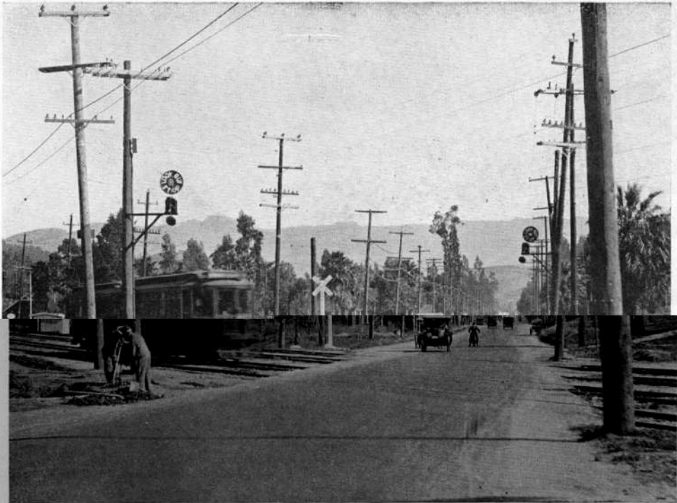
Double installation of 600-volt D. C. Magnetic Flagman, using power from trolley line, on Pacific Electric Railway four-track system at Huntington Boulevard, Los Angeles. Operation controlled by Trolley Brush Contacts, and Simplex Relays. There are over 1200 interurban train movements at this crossing per day. This railway has installed over 500 of our Magnetic Flagmen.
