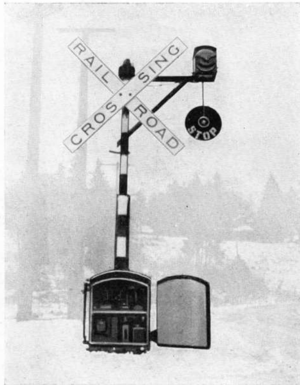
Installation of 3-volt D.C. Magnetic Flagman (two position, lower quadrant), on Northern Pacific R. R.
