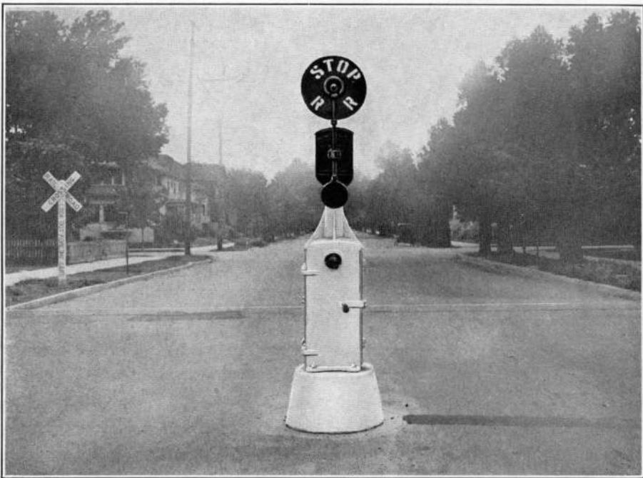
Center of Street Installation of Magnetic Flagman (two position, upper quadrant), on the Western Pacific Railroad, Sacramento, California.
