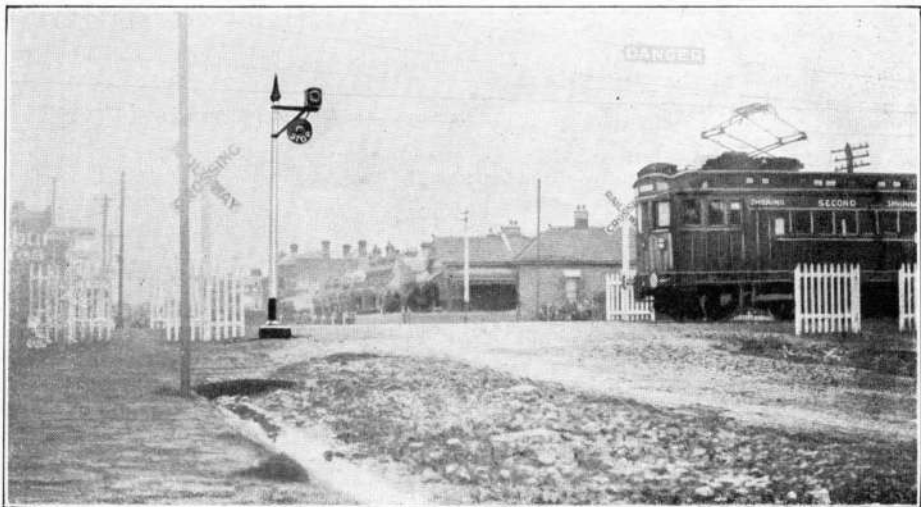
Installation of Magnetic Flagman (two position, lower quadrant), on Victorian Railways, at Melbourne, Australia.
