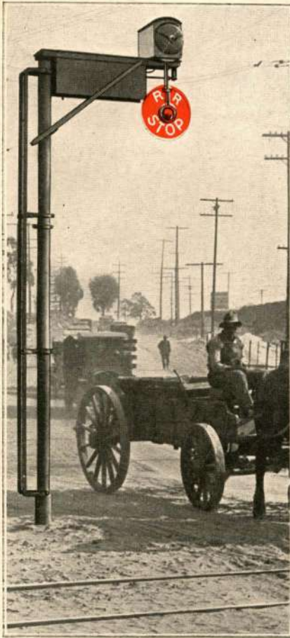
Magnetic Flagman together with "Out of Order" signal in normal operating position.
