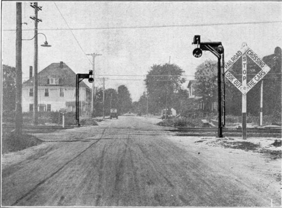
Two Position Magnetic Flagman together with "Out-of-Order" Auxiliary Signals in operation on the Long Island Railroad. Illustration shows Signal in normal operating position with "Out of Order" Banner concealed.
