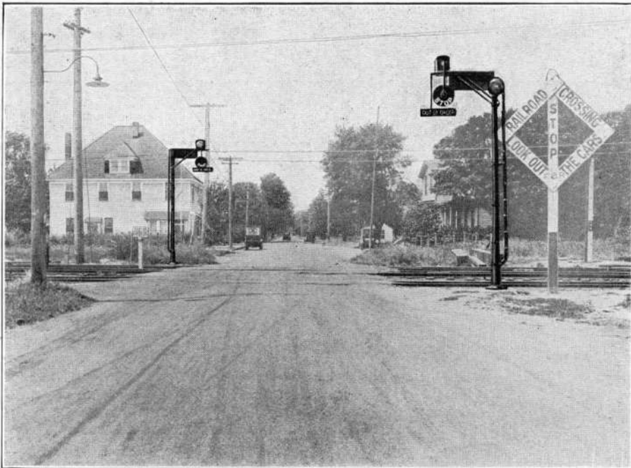
Illustrating same installation with "Out-of-Order" Banner dropped, indicating failure to operate from either electrical or mechanical causes.
