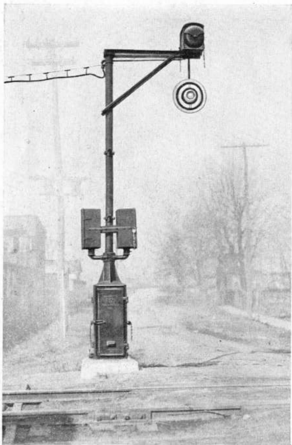
Installation of Magnetic Flagman (two position, lower quadrant), on Louisville & Nashville R. R., Lebanon, Ky.
