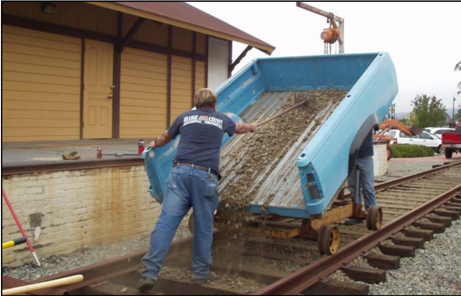
Ted VanKlaveren scrapes ballast from the Museum's dump car onto the display track.
