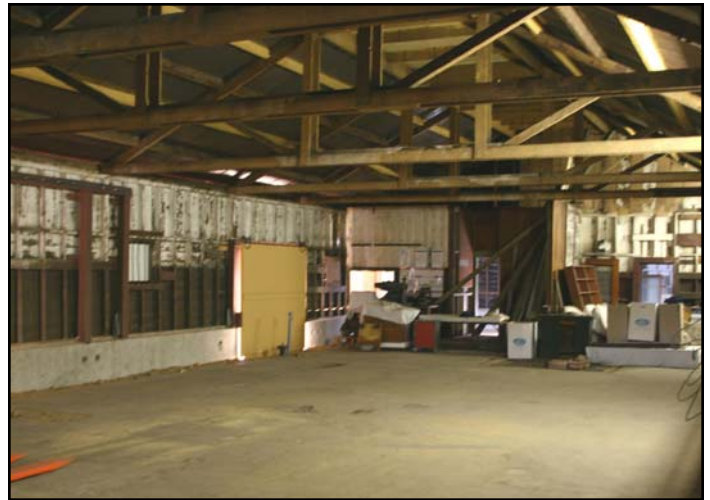
Freighthouse interior looking north.
