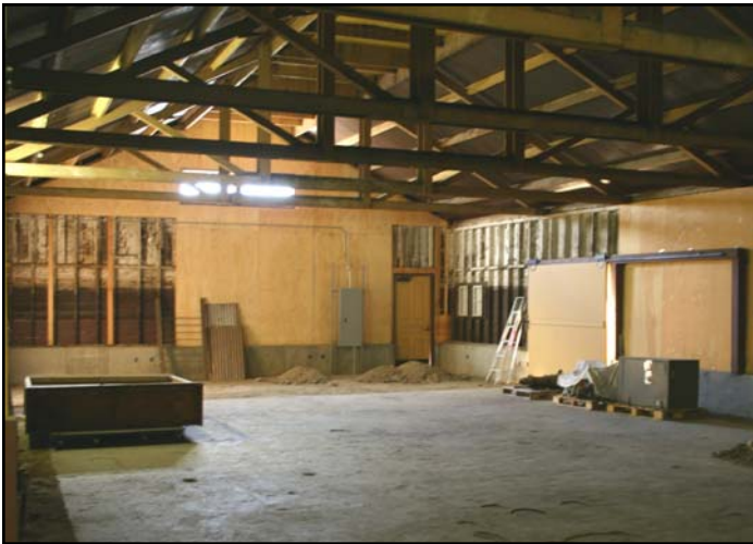
Freighthouse interior looking south.
